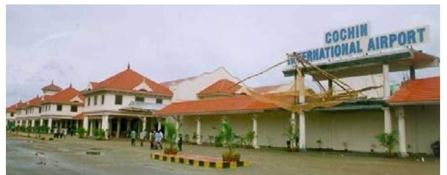
HUDCO-Funded Cochin International Airport
