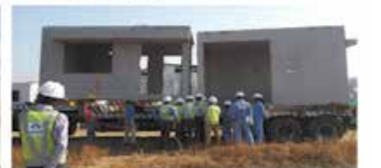
Transportation of Modules to Installation Site
