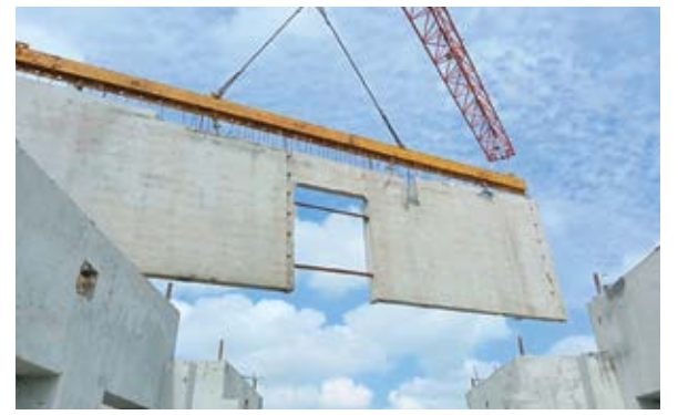
Fig.13: Placement of Walls
