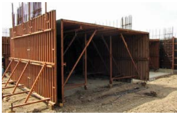
Fig.4: Installation of Tunnel Formwork
