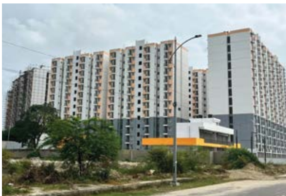
Fig.11: Completed buildings of Light House Project at Lucknow
