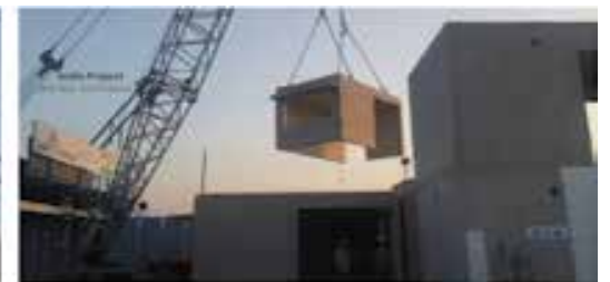
Casting & Stacking of Modules in the Casting Yard
