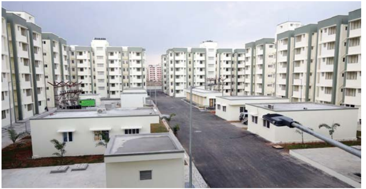
Fig.3: Completed Light House Project at Chennai
