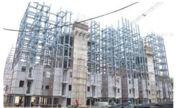
Fig.10: Placement of PVC Wall Form Panels in Steel Structure Frame
