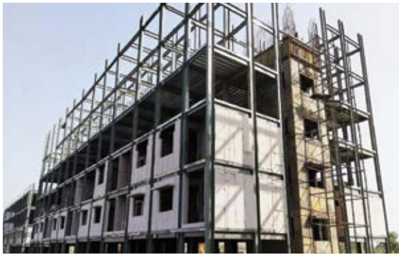
Fig.8: Placement of Prefabricated Sandwich Panels in Steel Structure Frame
