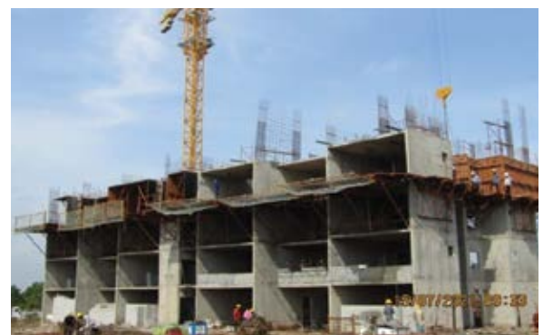
Fig.6: Tunnelform placing and casting of concrete
