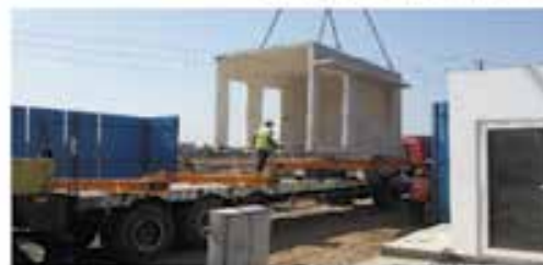
Transportation of Modules to Installation Site
