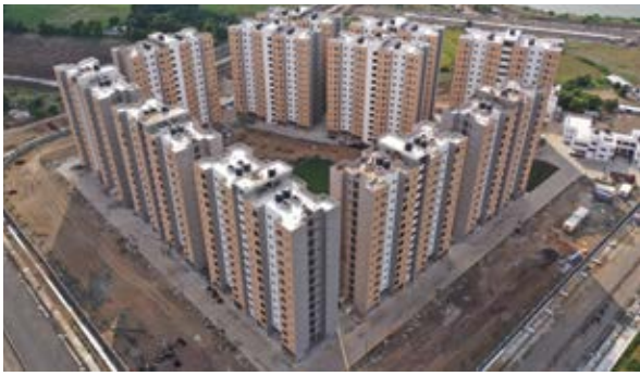
Fig.7: Completed Light House Project at Rajkot
