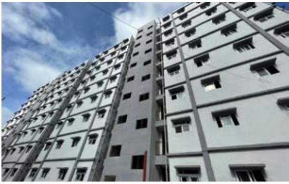
Fig.14: Finishing work in progress at Light House Project, Ranchi
