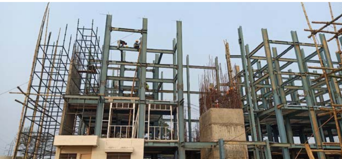
Fig.15: Placement of LGS frames in Steel Structure System
