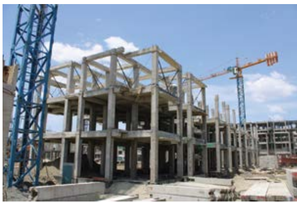
Fig.2: Beam - Column jointing
