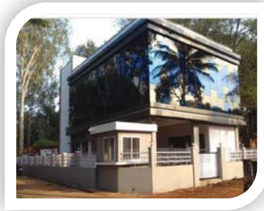
Command Control Center Belagavi
